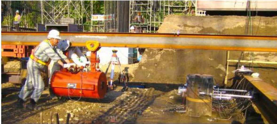
Photo 1. Loading and measuring devices in the Kiusu site.
